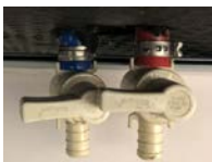
Low Point Drain Example
