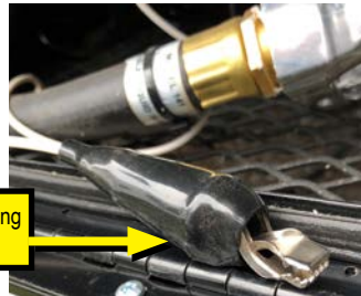
Grounding Clip Inside Fuel Station
