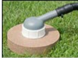
Dump Station Connection
