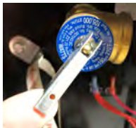
T&P Relief Valve Example
