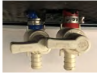
Low Point Drain Example
